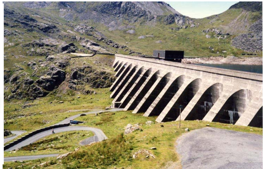
The upper reservoir of Ffestiniog pumped hydro storage system in Wales, UK.
